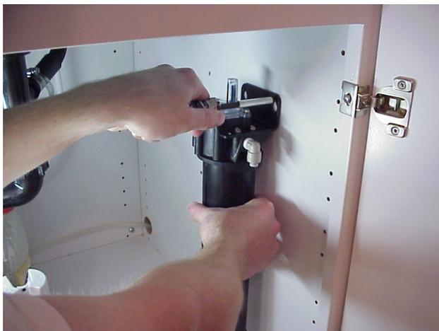
**Figure 5. Filter Bracket Installation**
