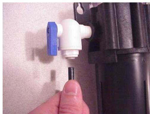
**Figure 8. Cold Water Supply Connection to Shutoff Valve**
