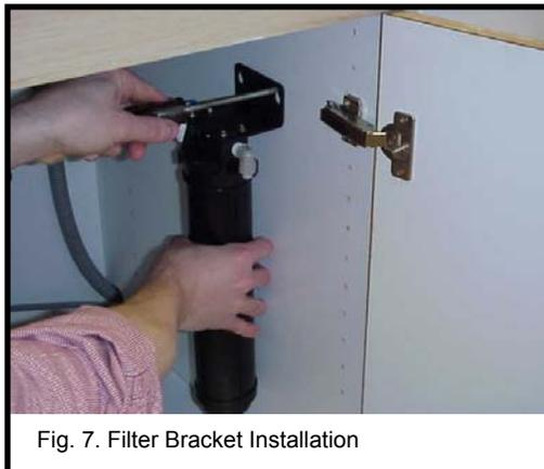
Fig. 7. Filter Bracket Installation
