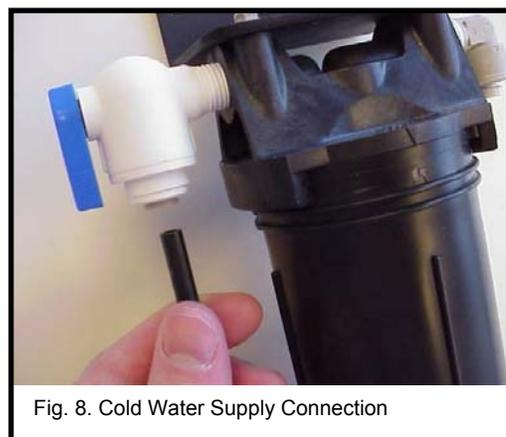
Fig. 8. Cold Water Supply Connection
