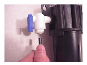
Figure 8. Cold Water Supply Connection to Shutoff Valve
