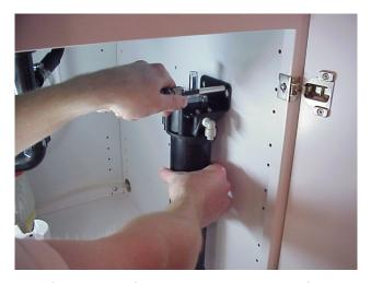
Figure 5. Filter Bracket Installation
