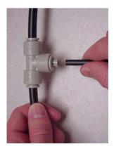
Figure 7. Cold Water Supply Connection to Tee Fitting
